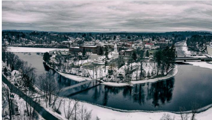
Swinging Bridge Skowhegan, ME. Over Kennebec River. From South side to Weston Island. Truss footbridge beyond, serving foot traffic to Water St, downtown.
