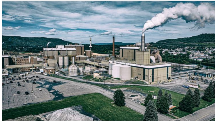
Twin Rivers Paper Factory, Edmundston, NB. Northern half of the international plant, spanning the St. John River between Madawaska, ME and Edmundston, NB. The Canadian portion, pictured, produces pulp and steam, piped across to the US portion which produces paper.
