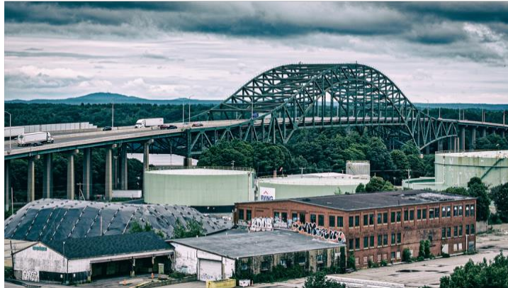
Piscataqua River Bridge over Portsmouth Harbor. A 'through arch bridge', built in 1972, completing Interstate I-95 between Portsmouth, NH and Kittery, ME.
