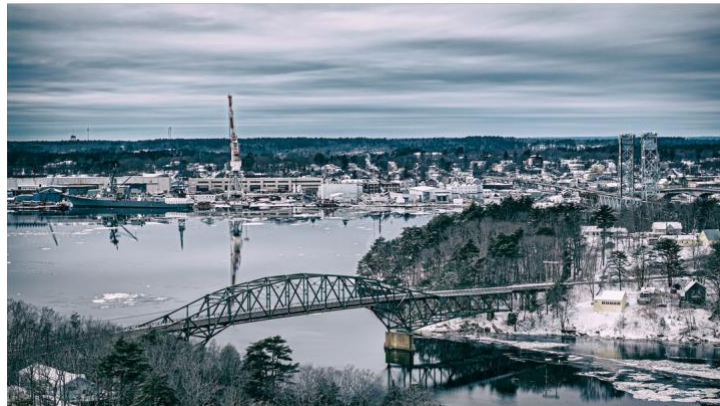
Max L Wilder Bridge, spanning Nequasset Brook, with Bath Iron Works in the background. Sagadahoc Bridge to the right, spanning the Kennebec River and Bath Harbor.
